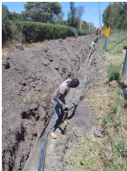
Laying of OD 110 water pipeline
