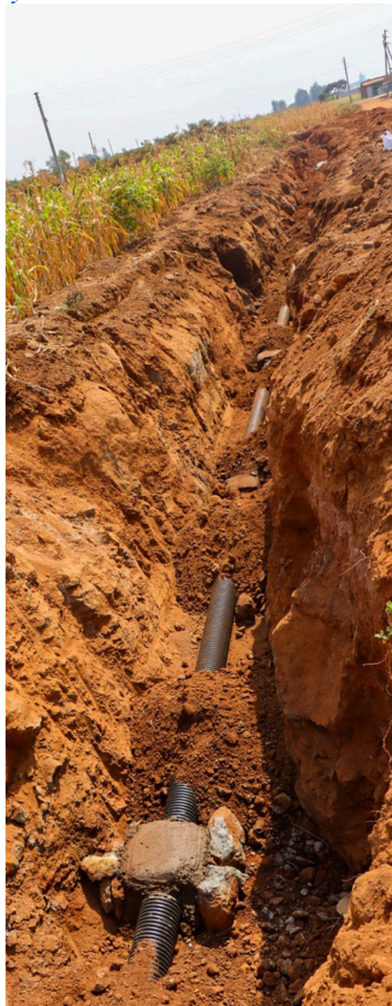
Back-filling of DN 200 Sewer Pipeline
