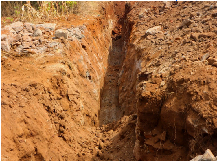
Excavation of trenches for DN 200 sewer pipeline
