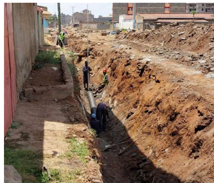
Excavation of trenches for laying of DN 300 sewer pipeline
