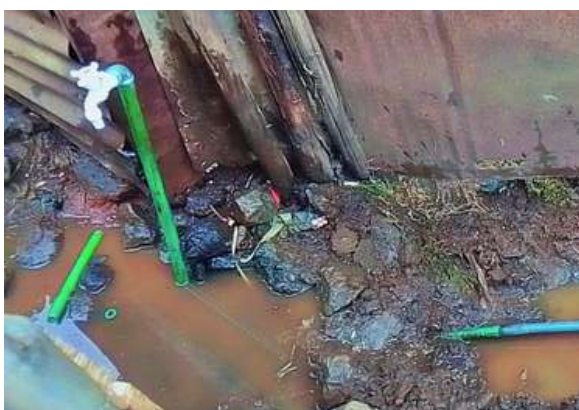
Trenching and laying of water Pipeline
