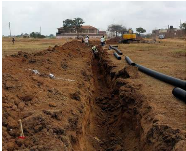
Excavation of trenches for DN200 sewer pipeline
